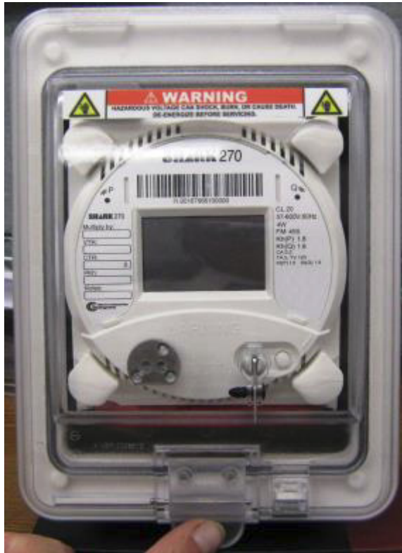
8:39: Closing the Switchboard Case
