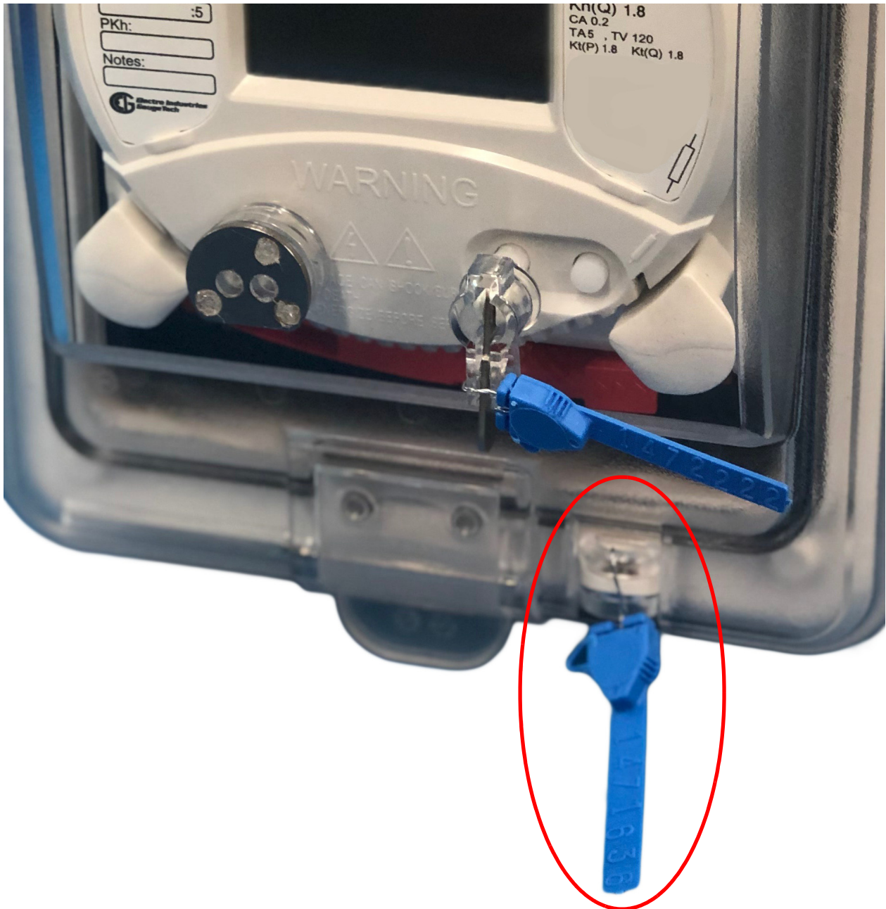
Figure 5.27: Sealing the Meter Cover - Switchboard Meter
